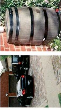
Installing permeable pavers (as opposed to asphalt or concrete) and rain barrels are two methods residents can adopt to help reduce runoff to storm sewers.
